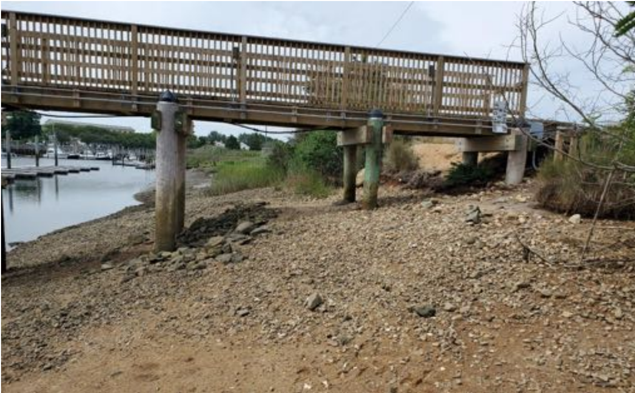
Photo 4. View of tidal flat north of existing Town pier facing south.
